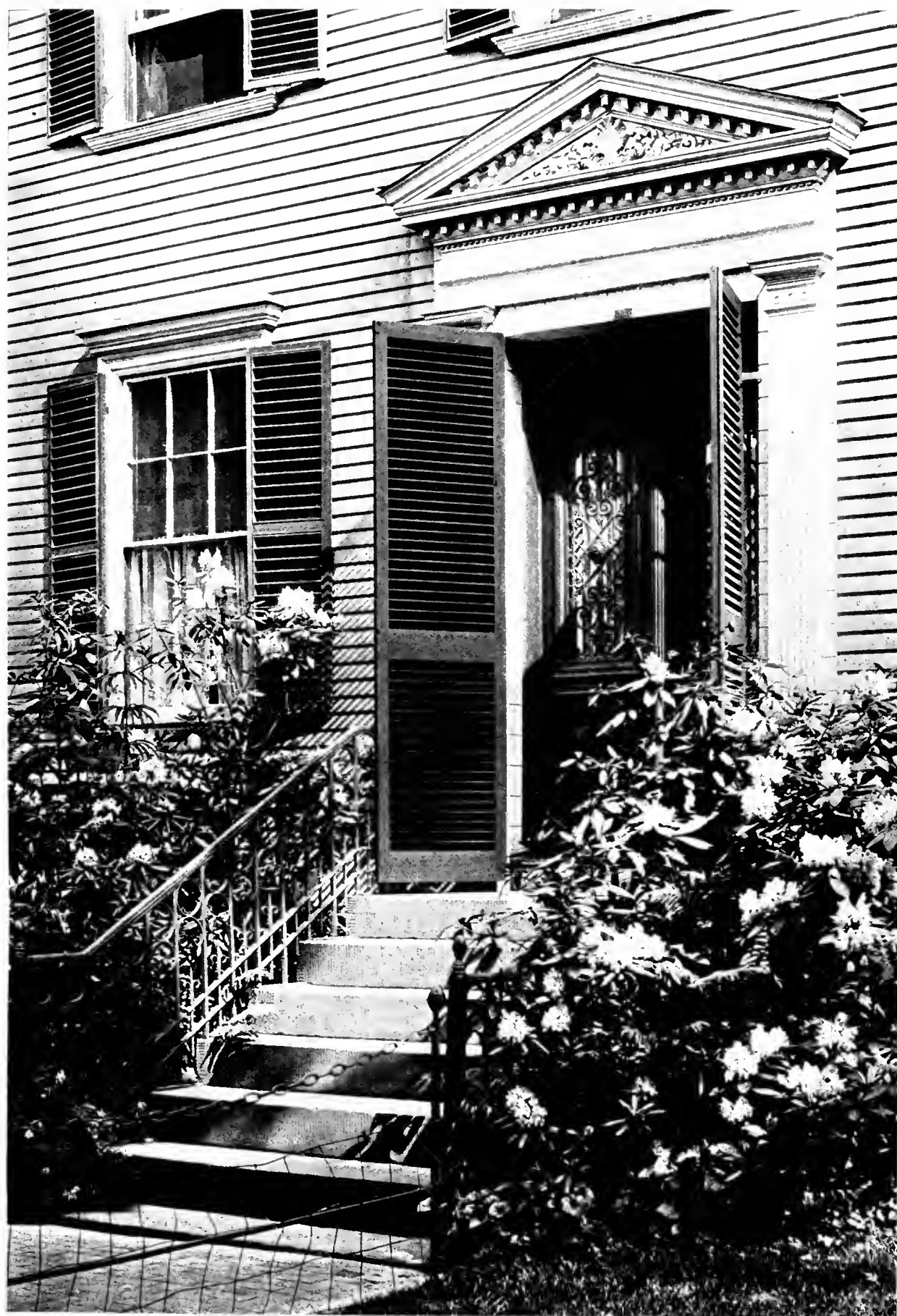
DOORWAY CABOT-ENDICOTT-LOW HOUSE, ESSEX STREET, SALEM, MASS. SAMUEL McINTIRE, ARCHITECT
